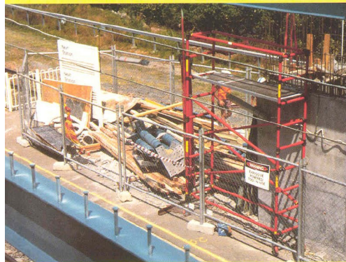
Rail platform widening
