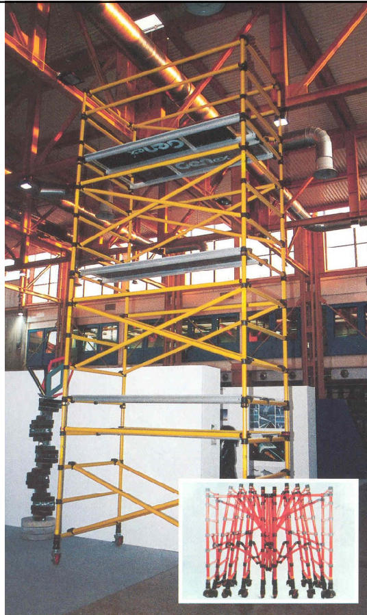
Assembly and maintenance of a thermic-conditioning
