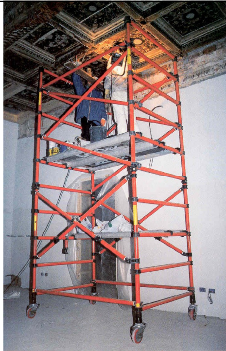
Restoration of a wooden ceiling (Bologna)
