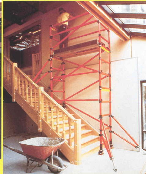
Tower on stairs with a difference in level of 1,5 m
