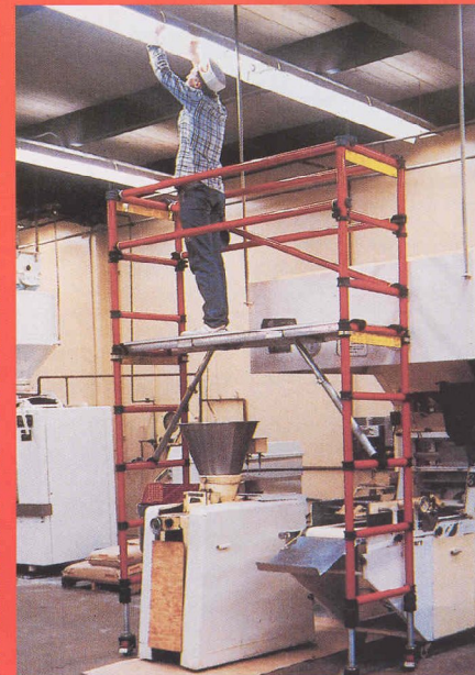
Assembly and maintenance of neon lights
