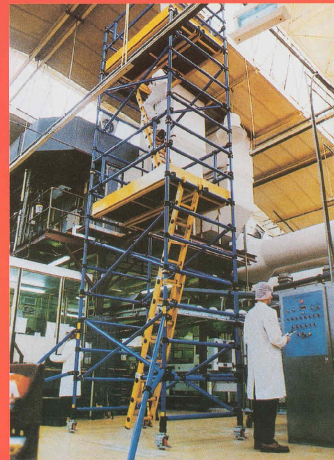
Inside maintenance with working system
