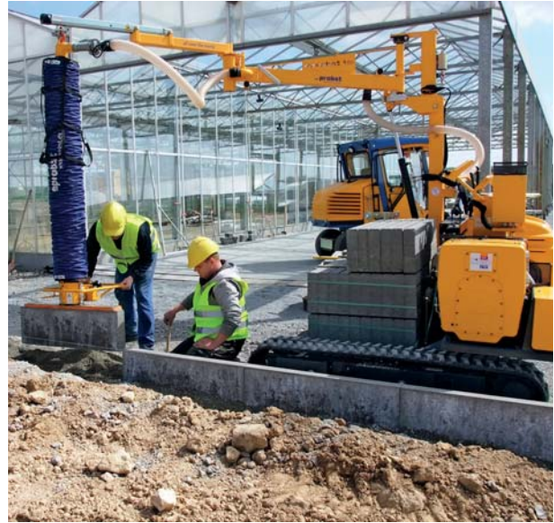
TRANSMOBIL TM Installation Carrier installing kerbs
