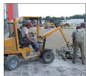
VM-203: Installation of large-format pavers
