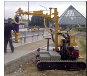
TRANSMOBIL TM Installation Carrier installing slabs
