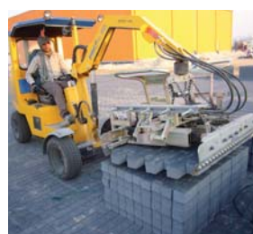
VM-203: Shifting rectangular pavers into running bond
