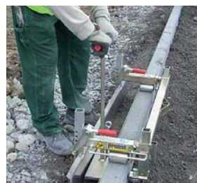
Slipform for Concrete Kerb Backfill GR-150
